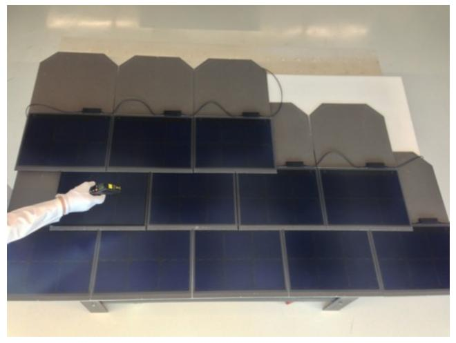
Each tile has a unique identification code and is recorded in a database with its ID, string number and position in the string. The tiles are identified individually with a gun at installation.
